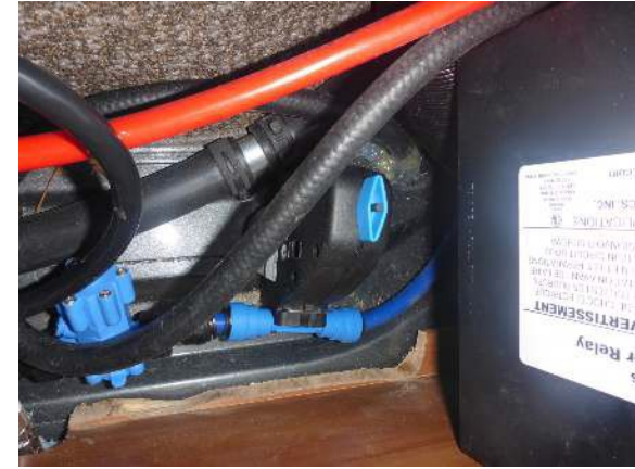
Frost control valve in tripped position
