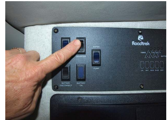
Picture 37.2 Inverter switch
