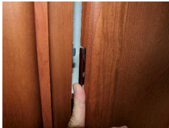
Hidden latch along edge of cabinet door
