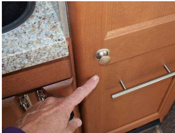
Pushbutton latch on cabinet door
