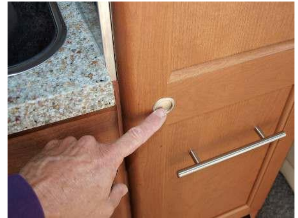
Locked pushbutton latch on cabinet door
