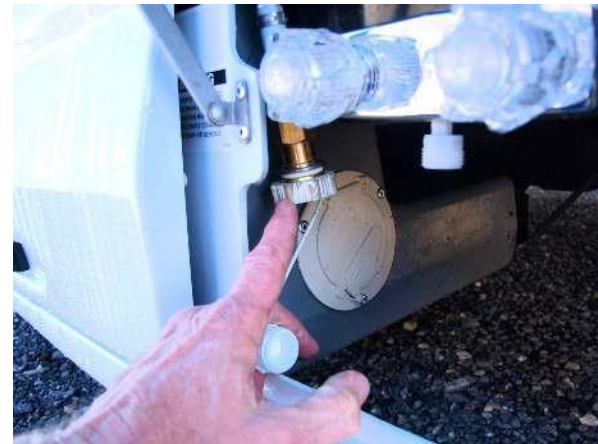
City water connection for hooking up to pressurized water
