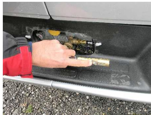
Propane pigtail with dust-cap removed and valve in open position
