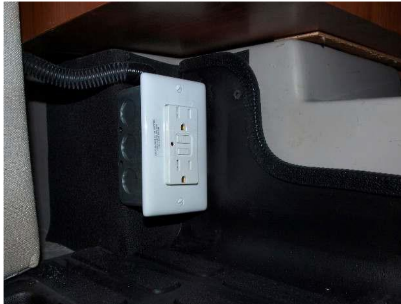
GFCI outlet under rear passenger side seat
