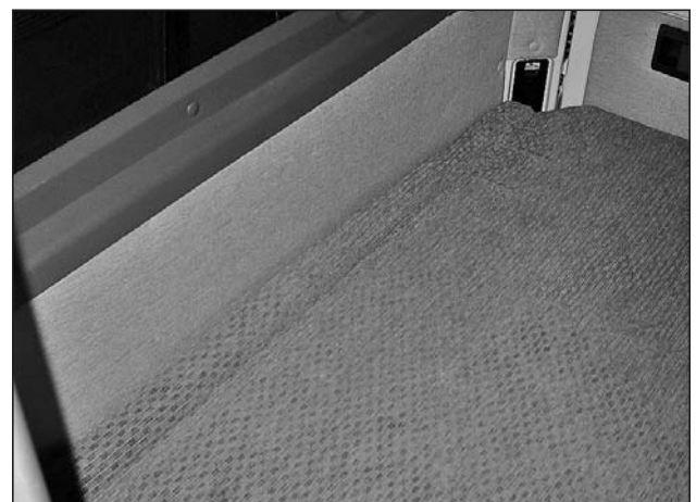
Picture B-P13: Placement of the filler cushion.
