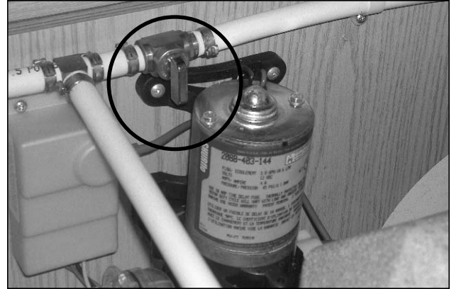
Picture G-P19: Hot water cutoff valve in closed position.
