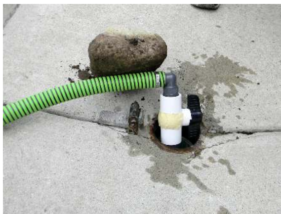
Use a convenient rock or other weight to hold hose down
