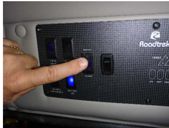
Water pump switch location on monitor panel
