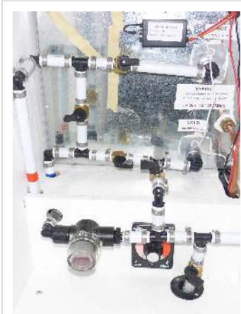
Tankless water heater inside cabinet - all valves are in normal operating position
