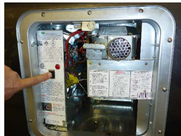
Turn off the water heater
