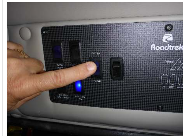
Water pump switch
