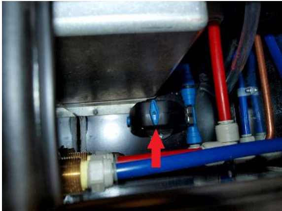
Alde valve in operating position
