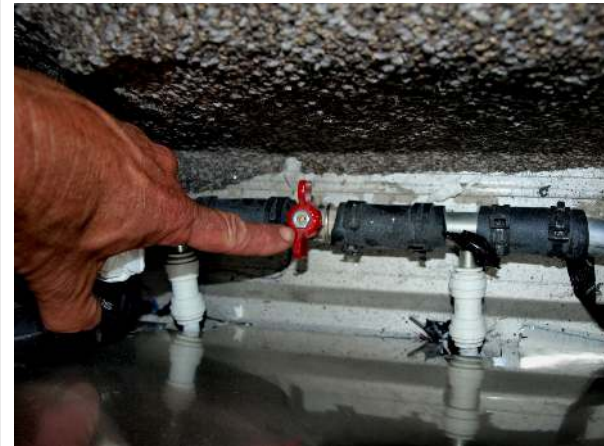
Alde floor bypass valve in full heat position (handle across the line)
