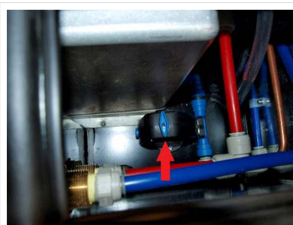
Alde valve in normal operating position
