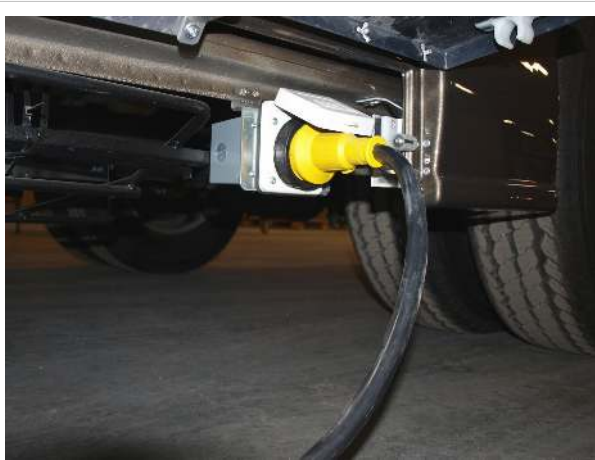
Shore power connection point
