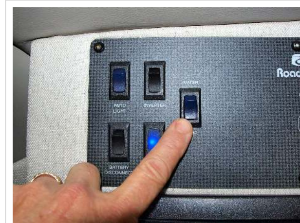
Water pump switch
