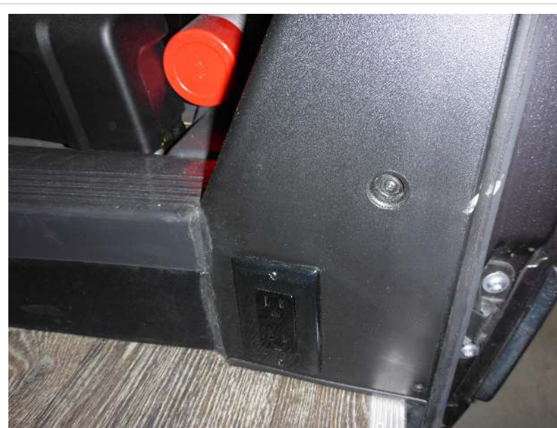
Outlet at side door
