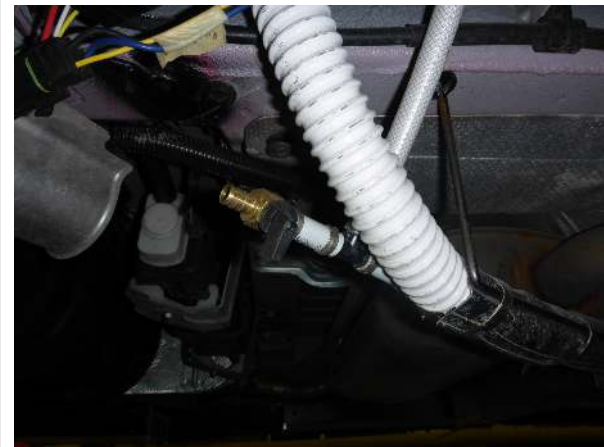
Fresh water tank drain, under driver's doorstep
