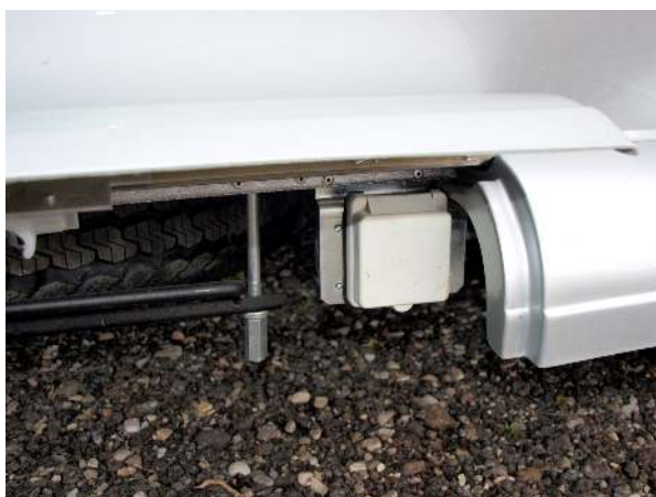
Shore power connection point
