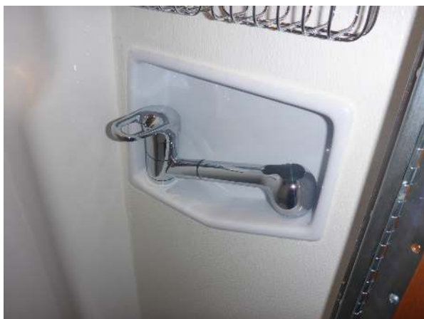
Shower hose stored
