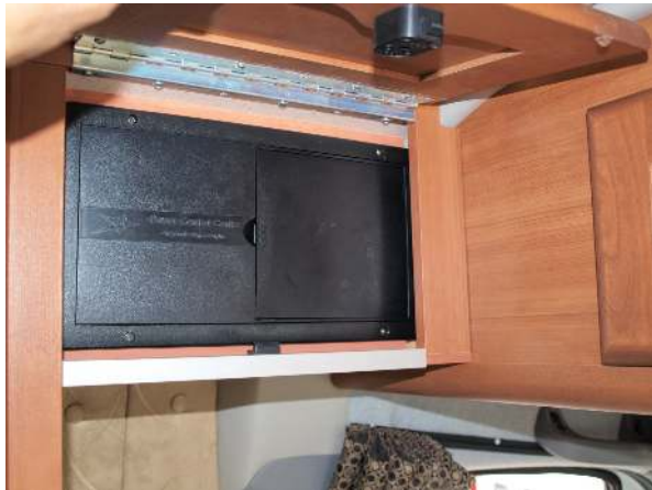
Agile power distribution panel location
