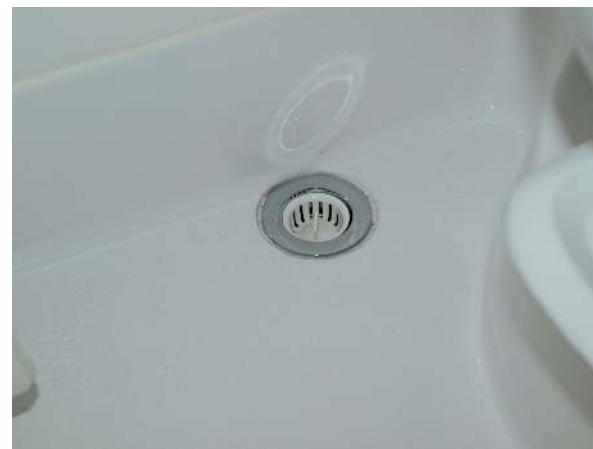
Shower floor drain plug
