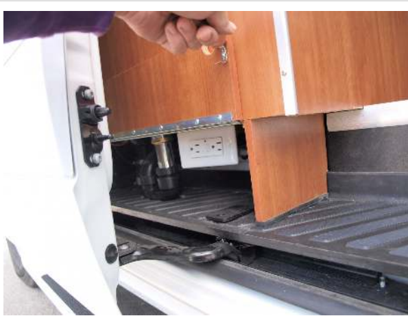
Access to city water valve
