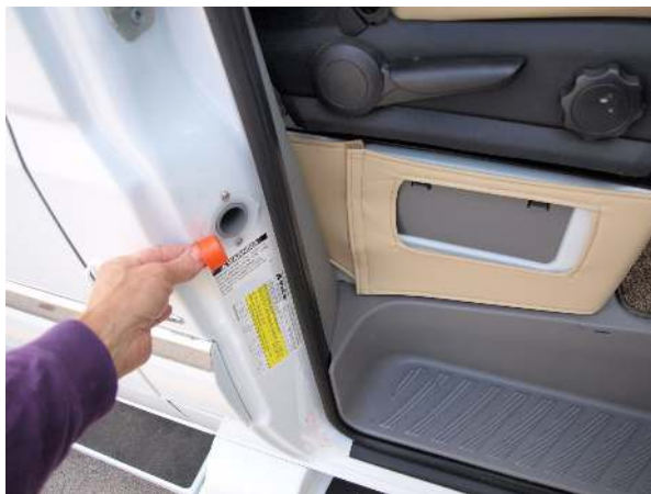
Fresh water gravity fill
