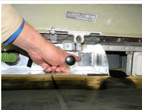
Cable TV connection location
