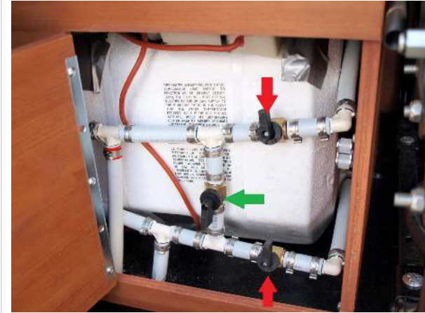
Water heater bypass valves in the bypass position, all handles vertical. Green means open, red closed.
