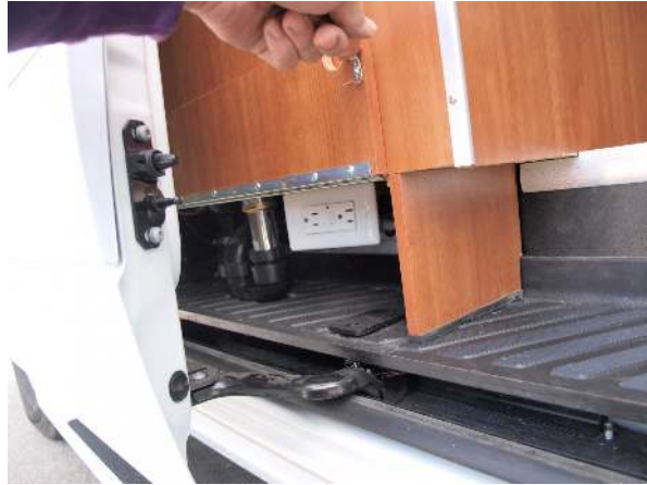
The city water valve is behind this access panel to the left of the side door opening
