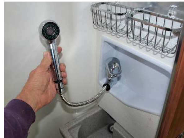
Shower hose extending from its storage location
