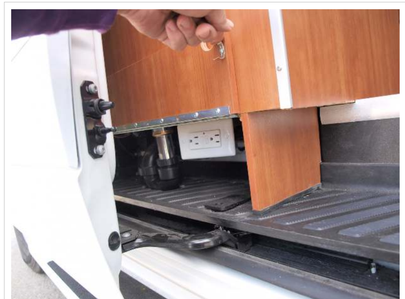
GFCI outlet behind rear seat
