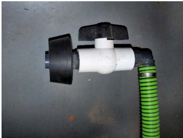
Doughnut installed on nozzle
