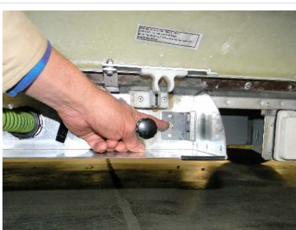
Cable TV connection location
