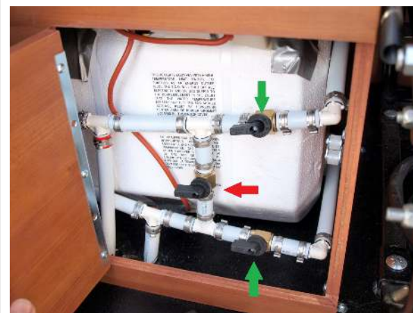
Water heater valves in normal position - green arrow means valve is open; red means shut. All handles point to the left.
