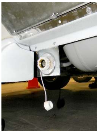
City water fill location
