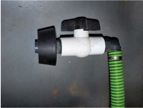
Rubber doughnut installed on nozzle
