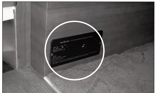
Picture F-P2b: Combination Carbon-Monoxide/Propane gas detector.
