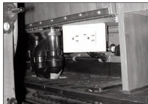
Picture E-P0B: 110V GFCI receptacle, (side entry door location).
