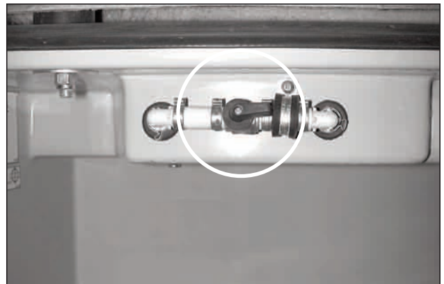
Picture G-P11: Open position of the city water tank fill valve.
