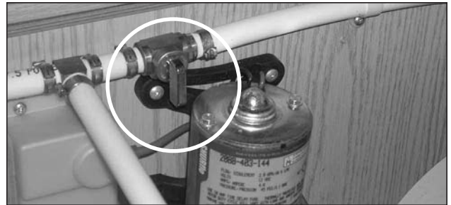
Picture G-P20: Hot water isolator valve in closed position.
