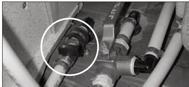
Picture G-P24: Interior tank transfer valve in closed position, (190 models).
