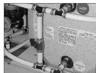
Picture G-P18A: Hot and cold water bypass valves, (170 and 190-Versatile models).
