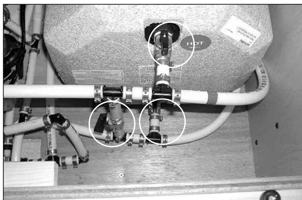
Picture G-P14: Normal mode water heater bypass valve positions.
