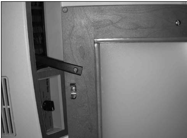
Picture B-P17: A/V cabinet door support in usage position.
