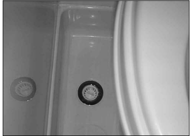
Picture B-P30: Location of bathroom shower drain.
