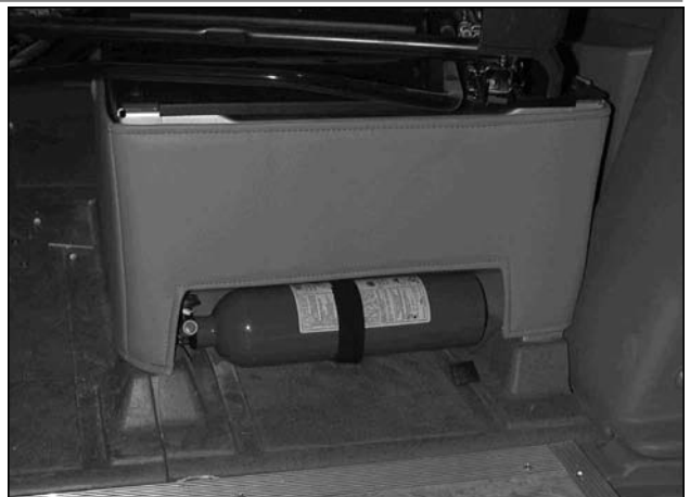
Picture F-P3: Fire Extinguisher location.
