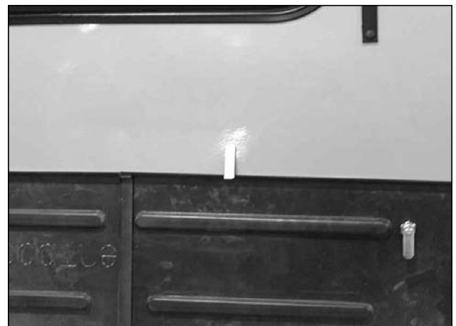
Picture B-P44: Rear storage area door hold up clip.
