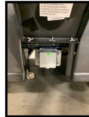
Picture 35.4 Shore power connection
