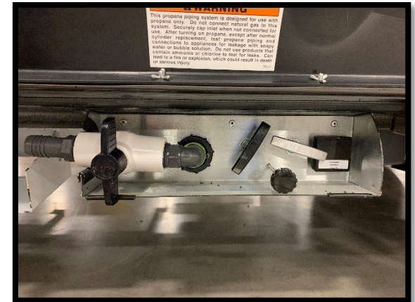
Wastewater hose, dump valves, pump cleaning knob, and CATV connection
