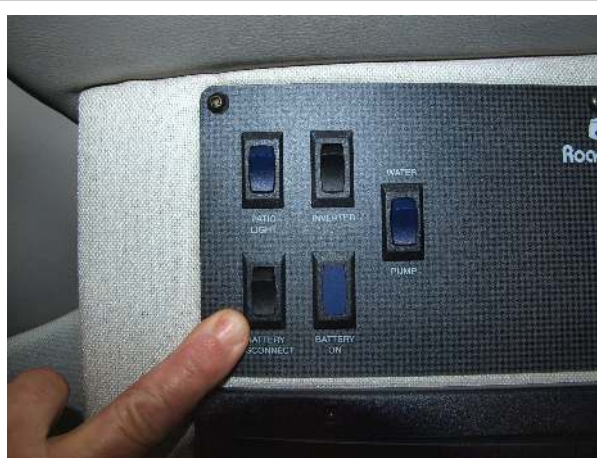
Battery disconnect switch
