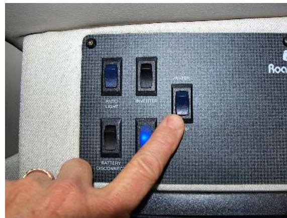
Water pump switch location on monitor panel
