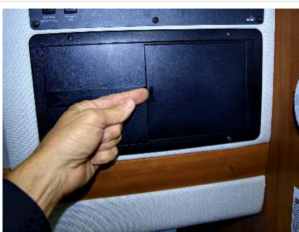
Breaker and fuse access
