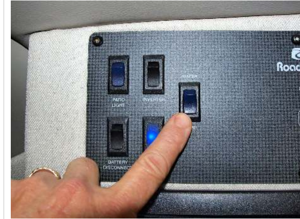
Water pump switch
