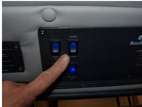
Water pump switch
