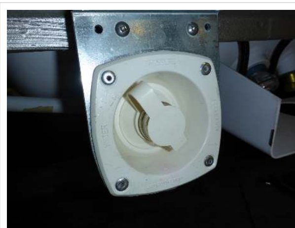
Built-in pressure regulator
