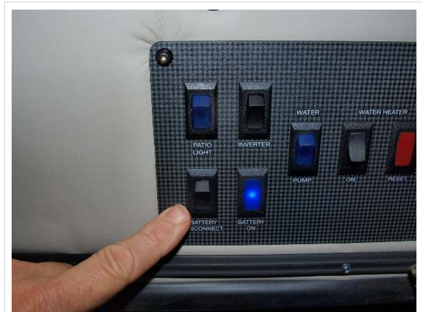
Battery disconnect switch on
