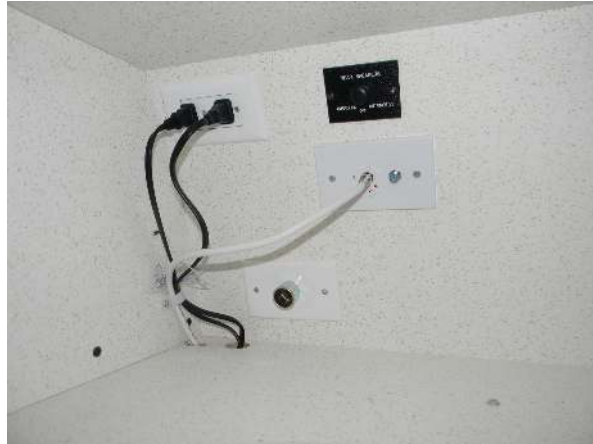
TV antenna switch and power injector
