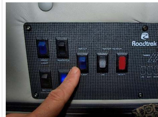
Water pump switch
