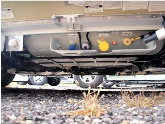
City water connection and propane tank
