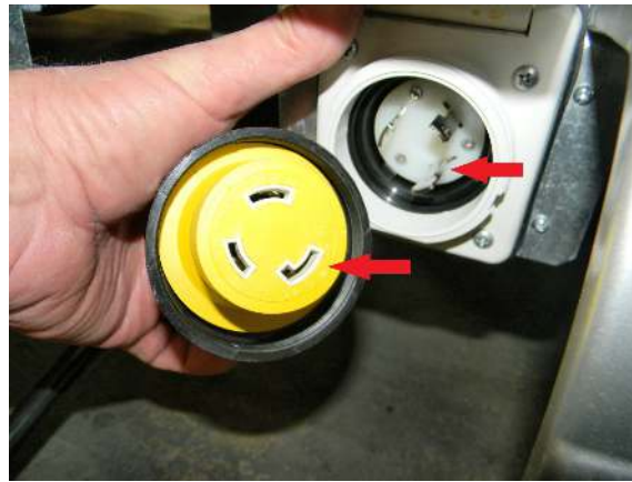
L-shaped prong on plug, and corresponding L-shaped hole in cord end
