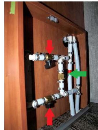
Water heater bypass valves in the bypass position. Green means open, red means closed.
