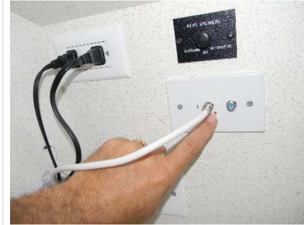
Switch between cable and TV
