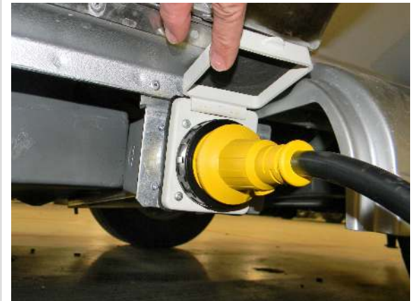
Attached shore power cord
