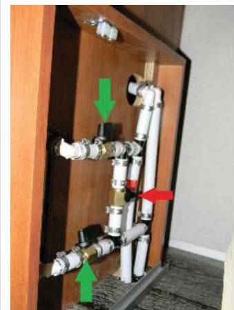
Water heater valves in normal position - green arrow means valve is open; red means shut.
