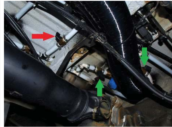
Webasto line valves in normal operating position
