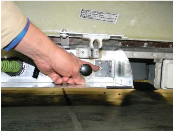
Cable TV connection location
