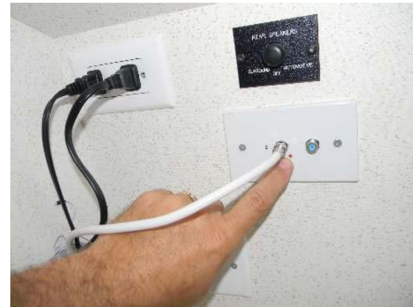
Switch between cable and TV
