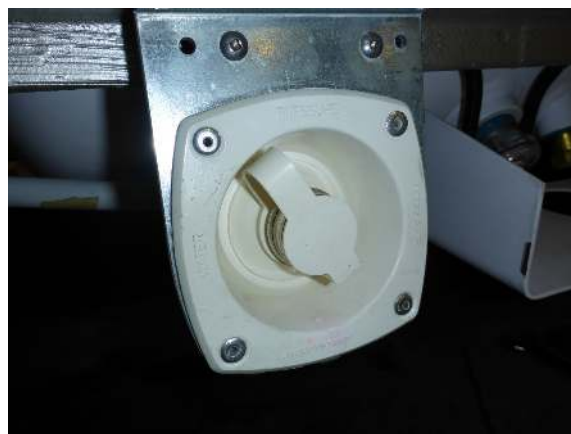
Built-in pressure regulator
