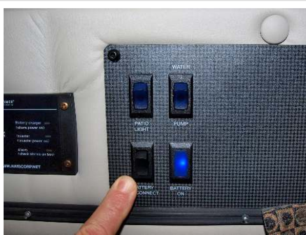
Battery disconnect switch
