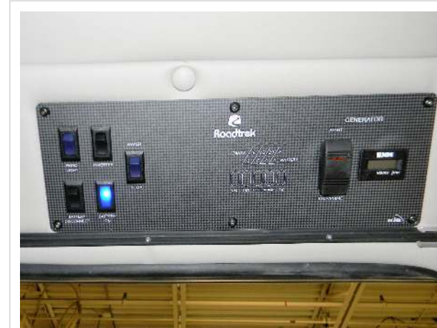
Monitor panel for units propane generator
