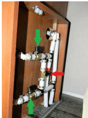
Bypass valves in normal position. Green means open, red means closed.
