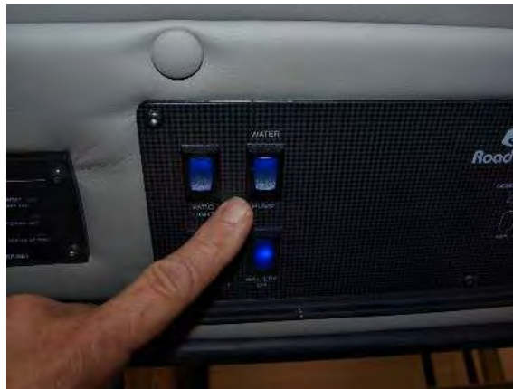
Water pump switch
