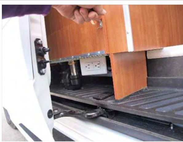
The city water valve is behind this access panel to the left of the side door opening
