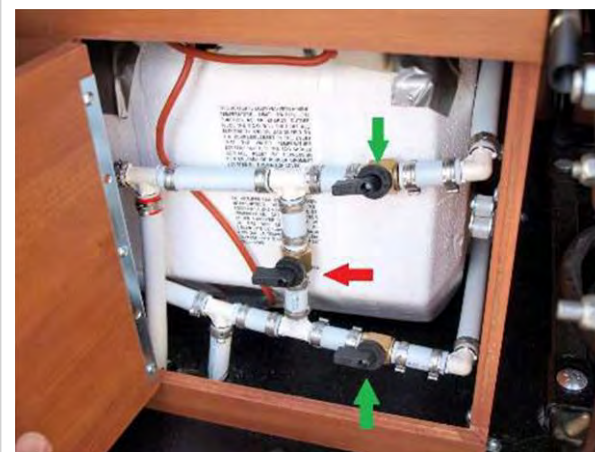
Water heater valves in normal position - green arrow means valve is open; red means shut. All handles point to the left.
