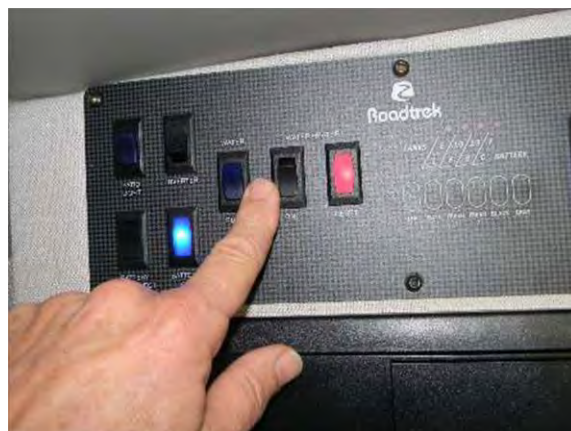
Water heater switch and red indicator light
