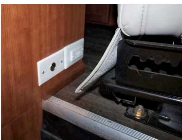
GFCI plug behind rear captain's seat
