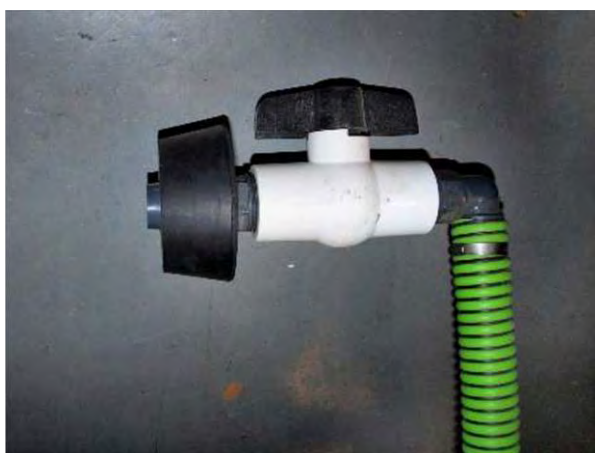
Rubber doughnut installed on nozzle
