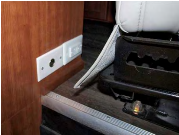
GFCI plug behind rear captain's seat
