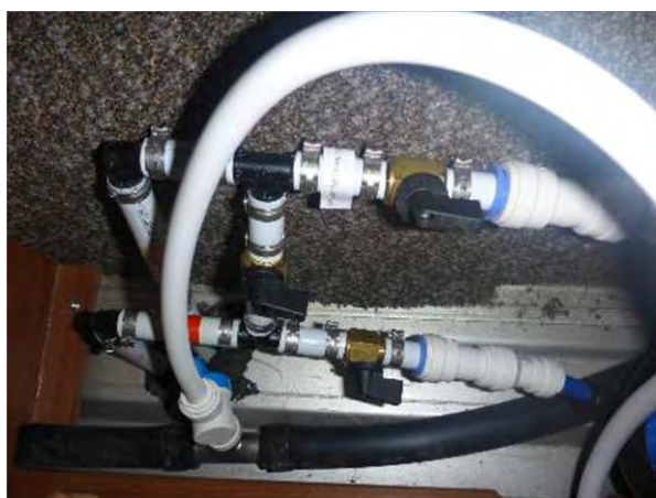
Alde bypass valves in normal operating position
