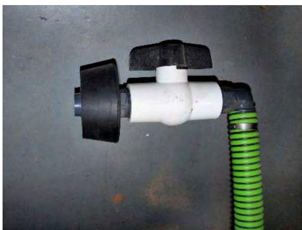
Rubber doughnut installed on nozzle
