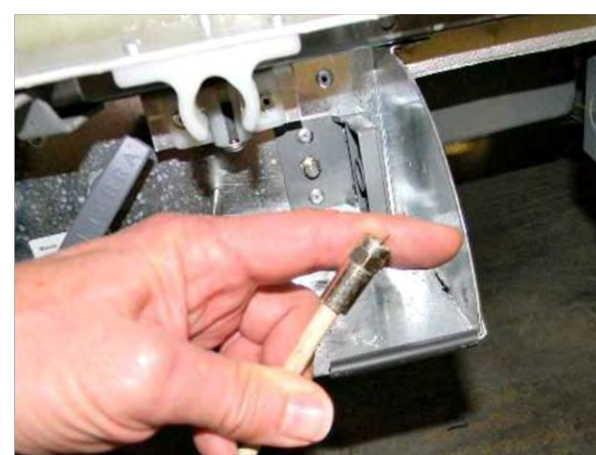
Coaxial TV connecting wire with screw-on end
