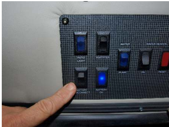
Battery disconnect switch
