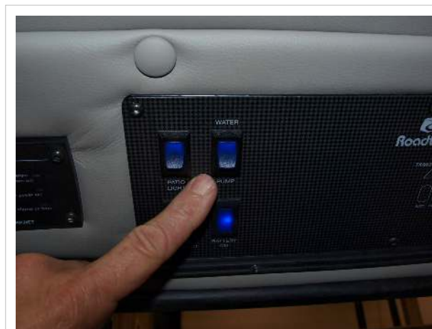
Water pump switch
