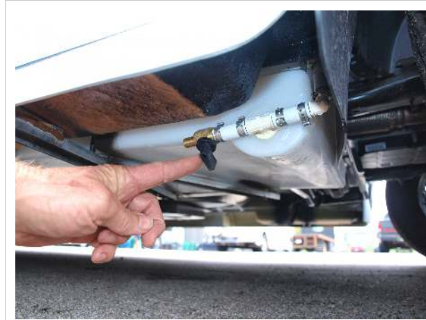
Drain for freshwater tank, beneath passenger doorstep
