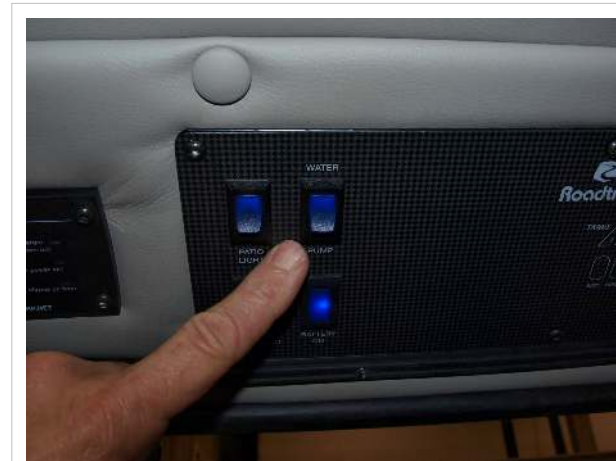
Water pump switch
