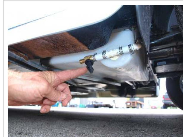
Fresh water tank drain valve
