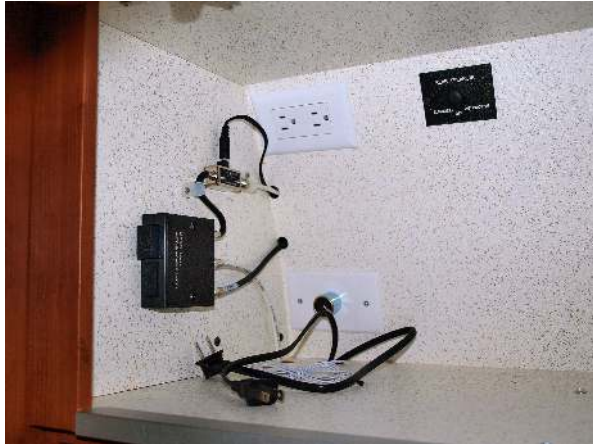
TV antenna switch and power injector
