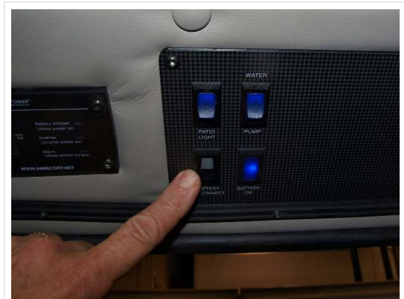
Battery disconnect switch
