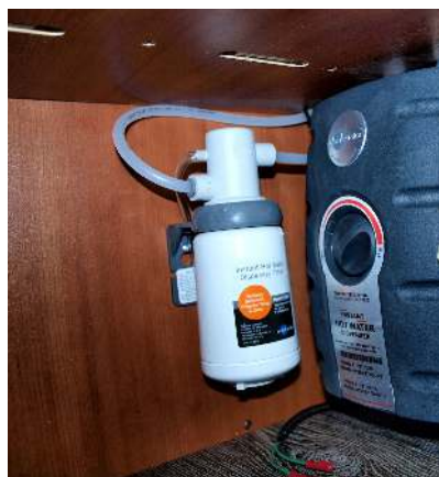
Filter for hot water dispenser, located in the galley cabinet
