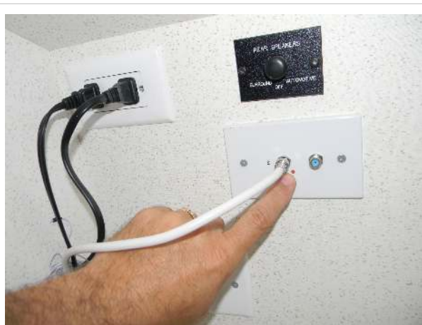
Antenna/cable AB switch set for antenna (top button)
