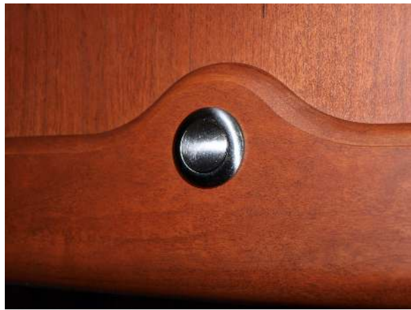
Pushbutton latch closed
