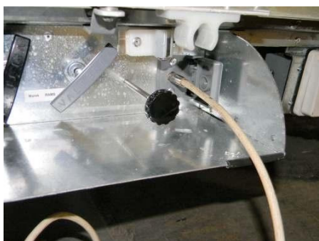
TV cable connected
