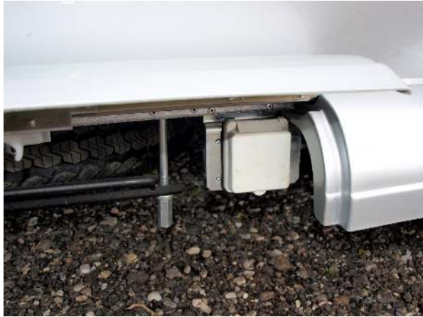
Shore power connection point
