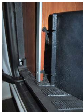
Screws holding plastic radiator cover on
