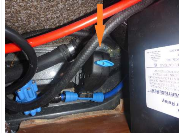
Frost protection valve in normal operating position
