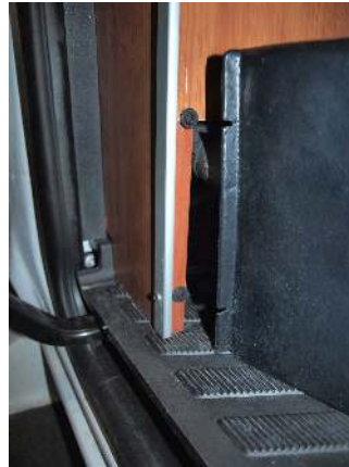
Screws holding plastic radiator cover on
