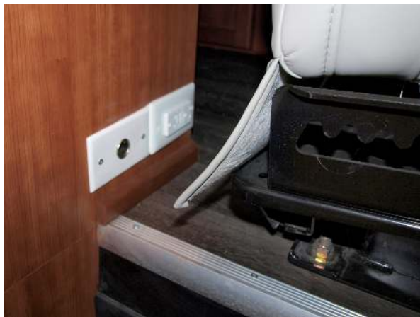
GFCI plug behind rear captain's seat
