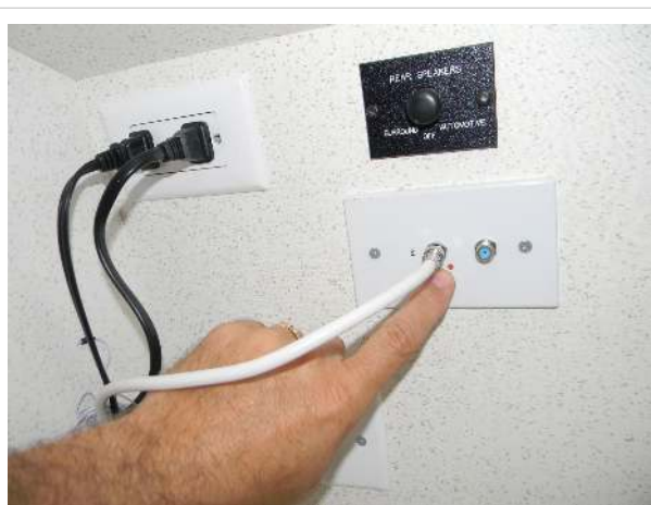
Antenna/cable switch (small white button on cover)
