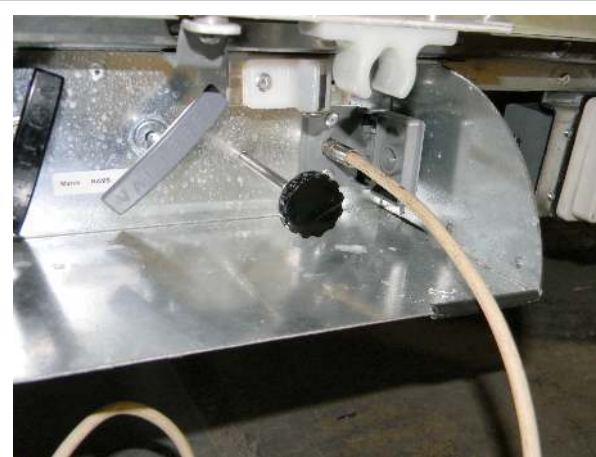
TV cable connected
