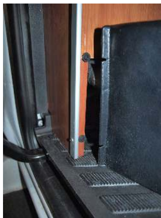
Screws holding plastic radiator cover on
