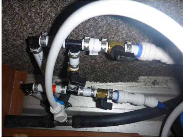
Alde bypass valves in normal operating position
