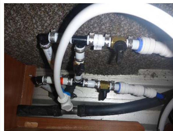
Valves turned to bypass position - all black handles vertical
