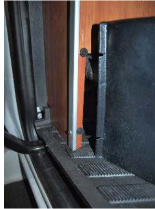
Screws holding plastic radiator cover on
