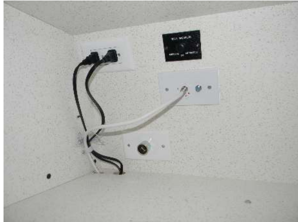
TV antenna switch and power injector
