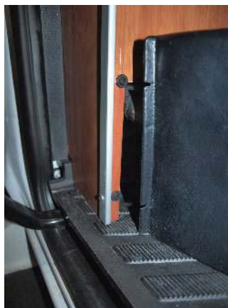
Screws holding plastic radiator cover on
