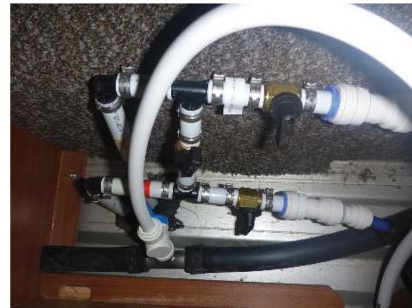
Valves turned to bypass position - all black handles vertical
