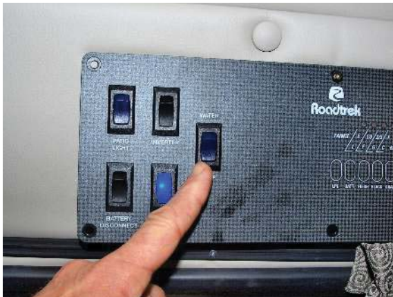
Water pump switch with standard inverter
