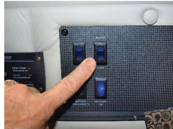
Water pump switch with 2500 watt inverter
