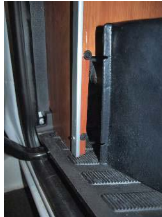
Screws holding plastic radiator cover on
