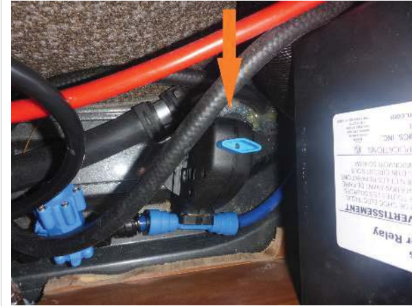
Frost protection valve in normal operating position
