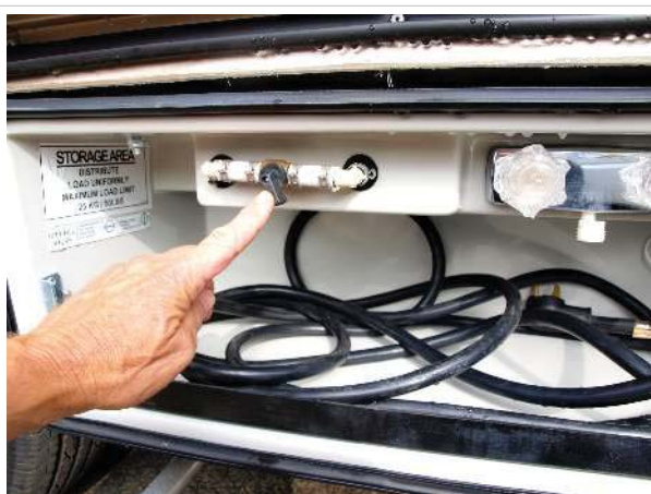
City water connection valve, shown closed
