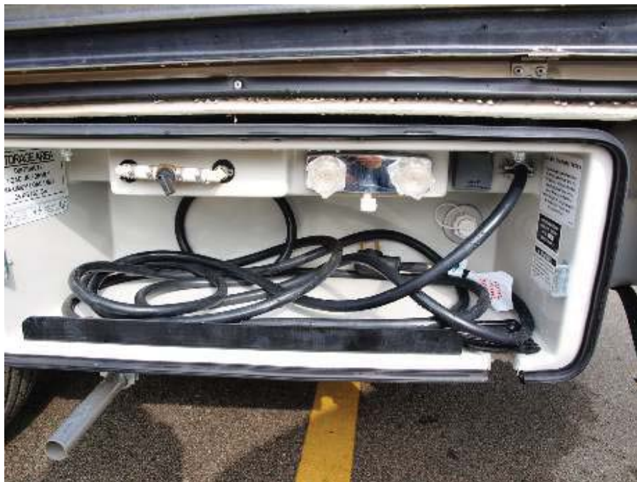
Driver's side rear compartment
