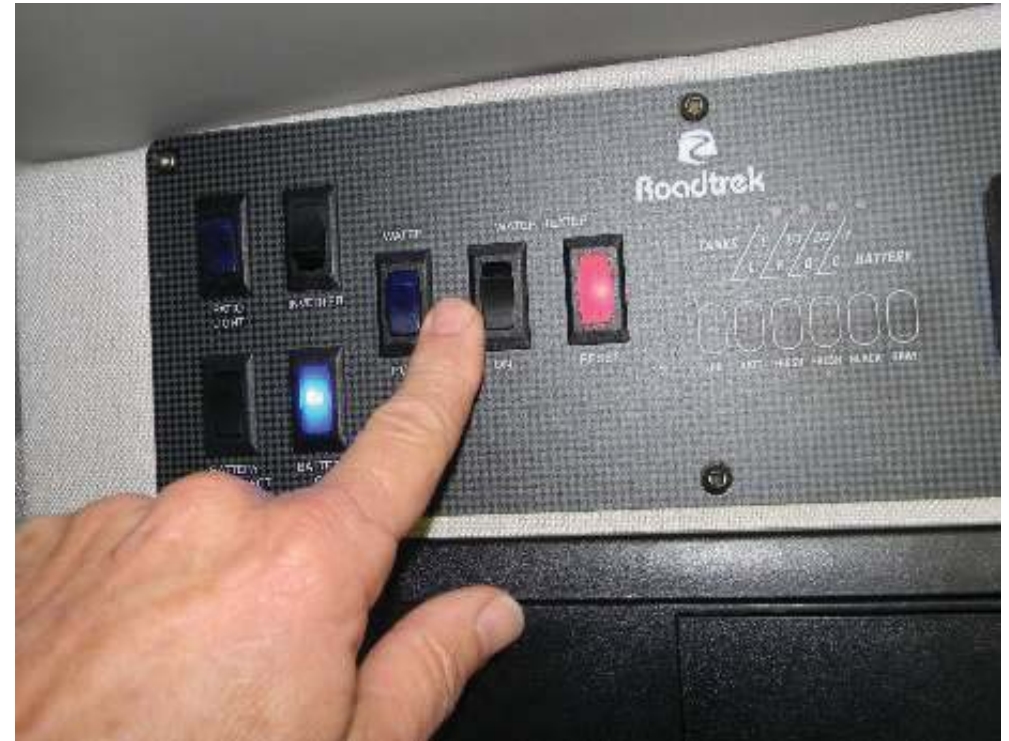
Water heater switch and red indicator light
