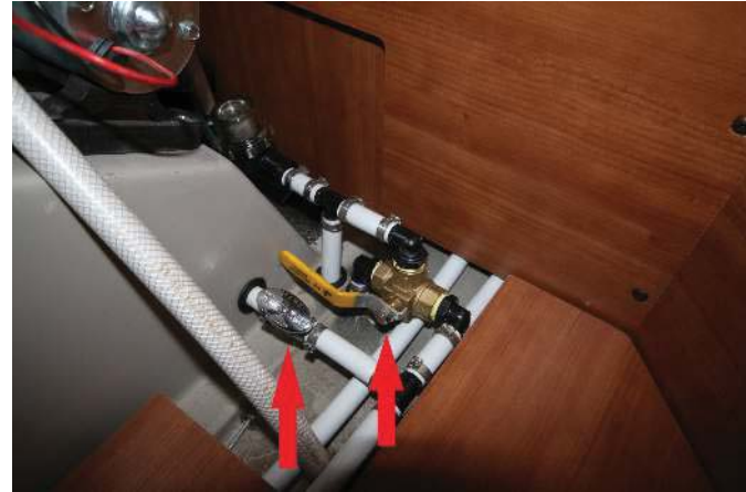
Tank isolator valve on the left in open or exterior position. Tank selector valve on the right in exterior tank position (colored plastic handle pointed to the driver's side of the Roadtrek).
