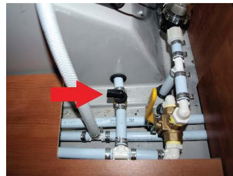
Tank isolator valve in closed position (black plastic handle pointed toward the back of the vehicle).
