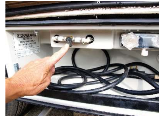
City water valve in closed position
