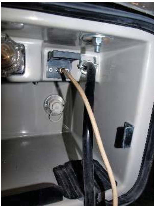
TV cable connected
