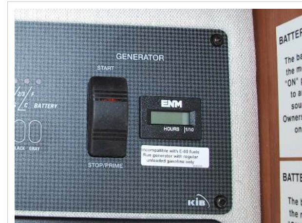
Generator switch and hour meter
