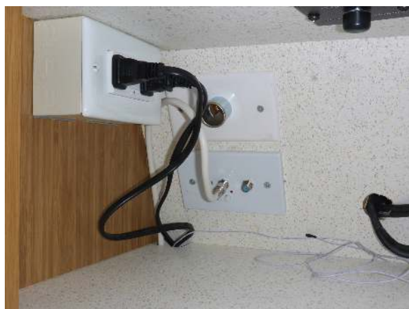
TV antenna switch and power injector
