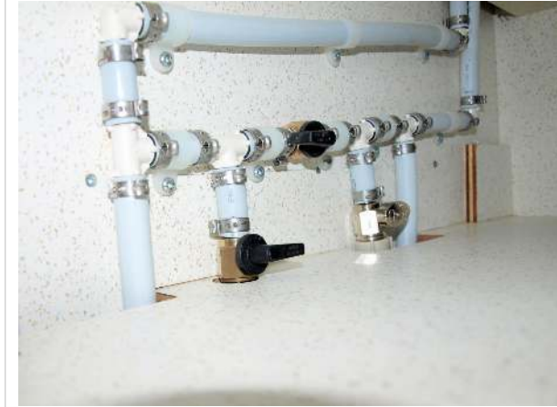
Water heater bypass valves in the bypass position
