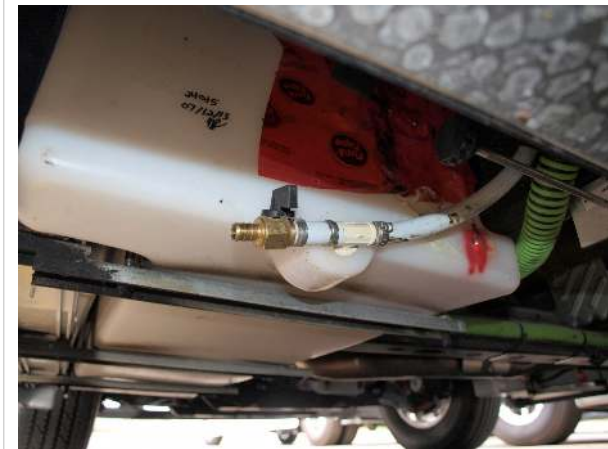
Exterior tank drain, under driver's door step
