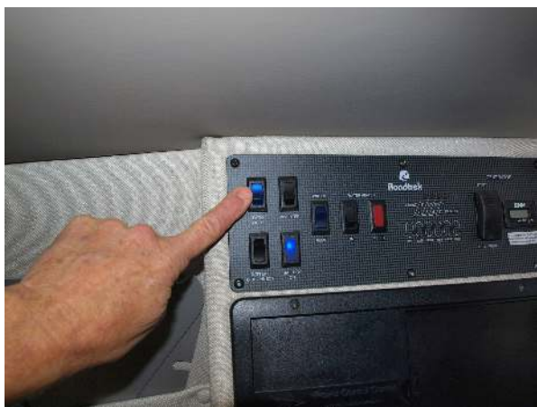
Patio light switch
