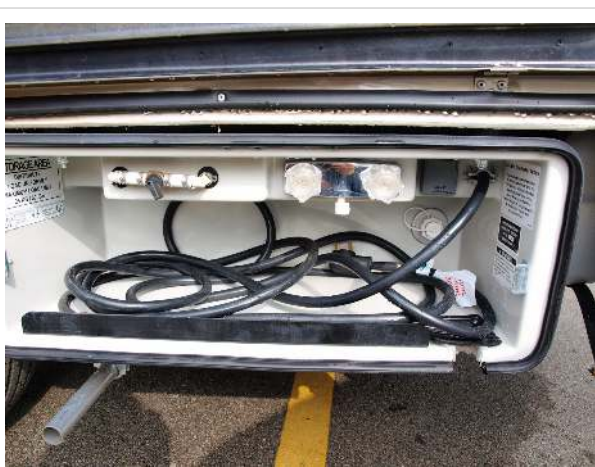
Driver's side rear compartment
