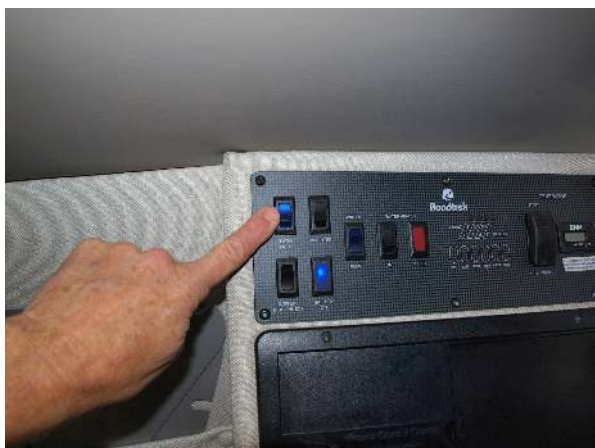
Patio light switch
