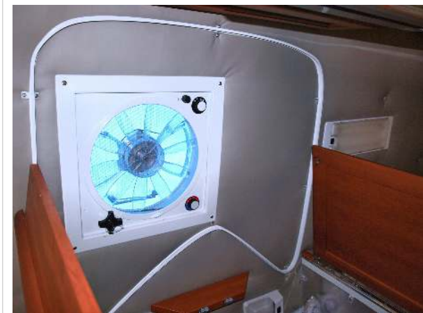
Shower curtain track
