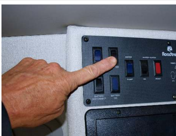
Inverter switch with standard 750 watt inverter
