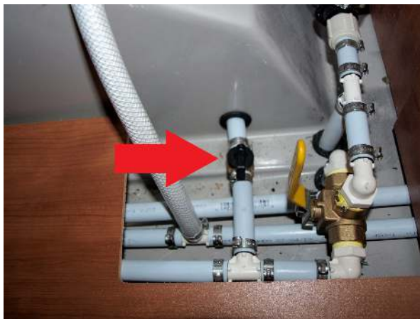
Tank isolator valve, shown in open position (black plastic handle pointed along the water line)
