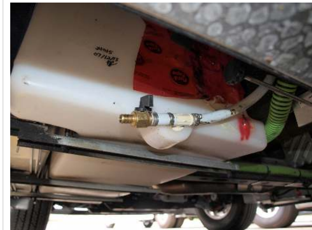
Exterior tank drain, under driver's door step
