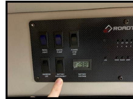
Battery Disconnect Switch 43.3
