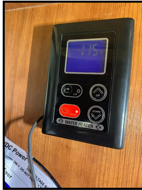
26.3 Water heater control panel
