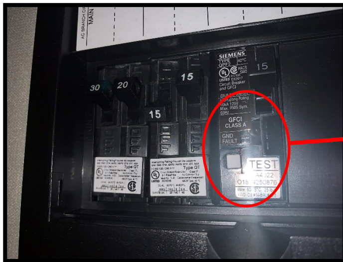
GFCI located on the fuse panel above the driver's seat
